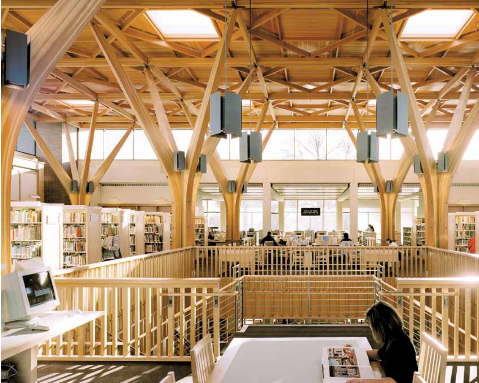
Local wood plays significant structural and aesthetic roles in the Beaverton library. (Photo courtesy of THA Architecture, Portland)
